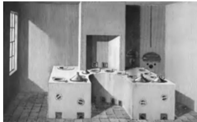
Fig 2. Perspective view of a kitchen fire-place in the house of Baron Lerchenfeld in Munich designed by Count Rumford, ca. 1870
